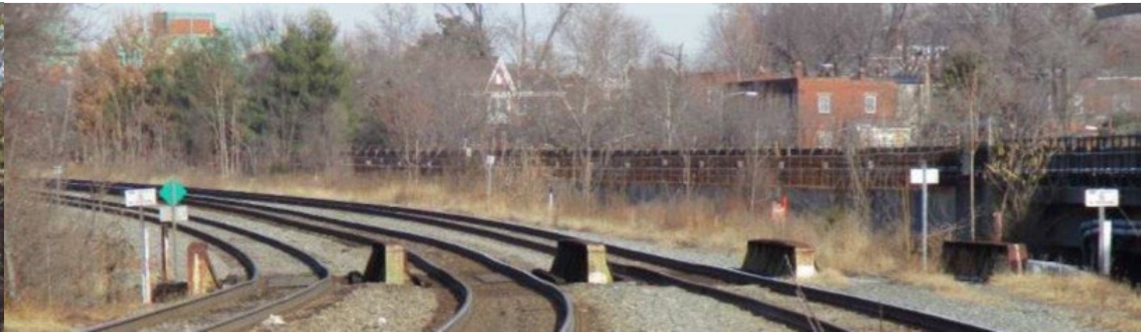
Rail Bridges over Commonwealth Ave, facing North
