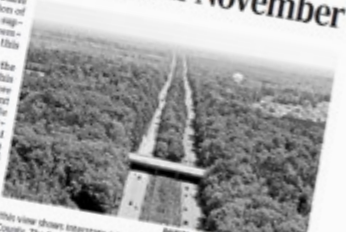
This view shows Interstate 64 near the Bottoms Bridge exit in New Kent County. The first I-64 widening work will carve away at the median east for Route 219 and Providence Forge.
