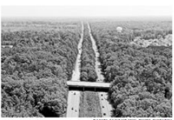
This view shows Interstate 64 near the Bottoms Bridge exit in New Kent County. The first 1-64 widening work will carve away at the median between mile 205, by the Bottoms Bridge exit, to mile 215, just east of the exit for Route 155 and Providence Forge.
